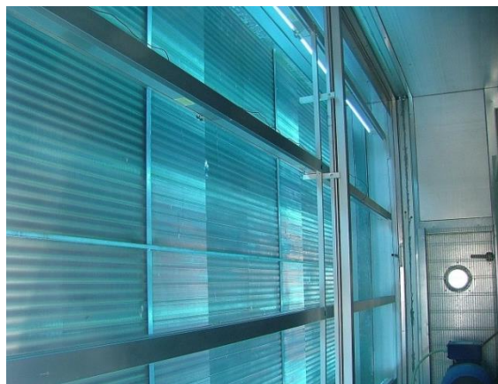
Figure 1. UVGI System Design
