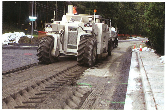
Reclaimer processing FDR (photo: Harris & Associates)
