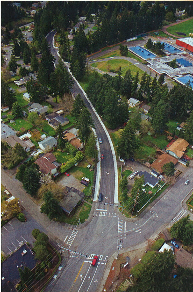
Aerial photo of Olympic View Drive, Phase 1, at completion (photo: Harris & Associates)
