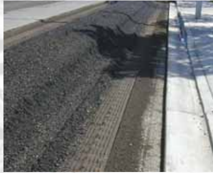
(Above Left) Deteriorated street in need of repair. (Above Middle) Cold In-Place Recycled windrow ready to be picked up and paved. (Above Right) Finish capped "renewed" road.
