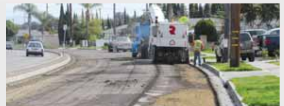
(Top) Cold In-Place Recycling train.
